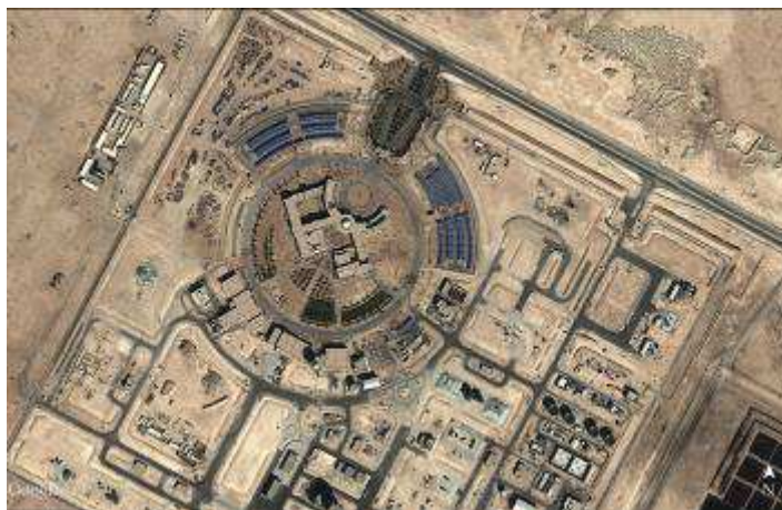
The Ras Laffan Emergency & Safety College project © Google Earth Imagery © 2013 Digital Globe. January 17, 2013. 25.883702, 51.431839
