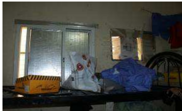
Hole in the wall where an air conditioner should be installed. Camp in Doha's Industrial Area, October 2012
