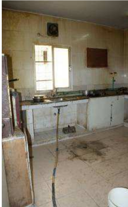
The downstairs kitchen at the PCSI workers' accommodation, October 2012. There is a boarded up hole where an air conditioning unit is meant to be installed, and drainage problems mean that the floor is partially flooded © Amnesty International
